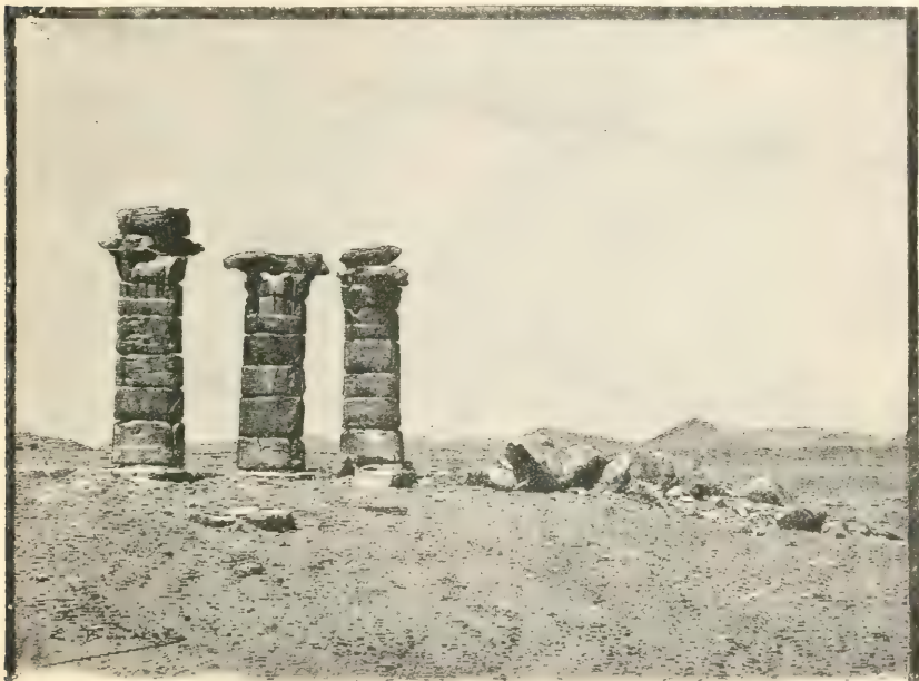
THE THREE STANDING COLUMNS OF THE TEMPLE OF SESEBI. 1
